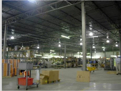
Representation of the area space. objects: Beams, ceiling structure, crates
