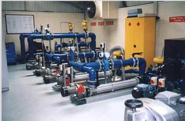
Pumping station. objects: Pumps, pipes, controls, ceiling lamps
